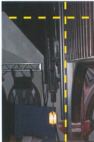
Deflection of the truss corners resulting from inadequate connection between the truss sections is seen in the corbel ends, which have dropped 3-4". Note degree out of plumb.
