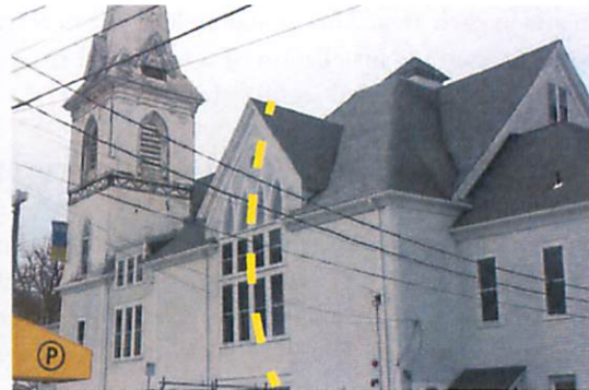
Bowing of window wall at the south transept is exacerbated by the framing deficits at the roof and corbel trusses. The wall is 6"-9" out of plumb.
