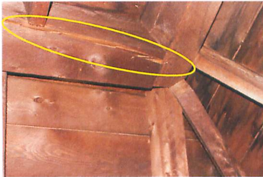
Split at roof collar beam at apex of main hip roof.
