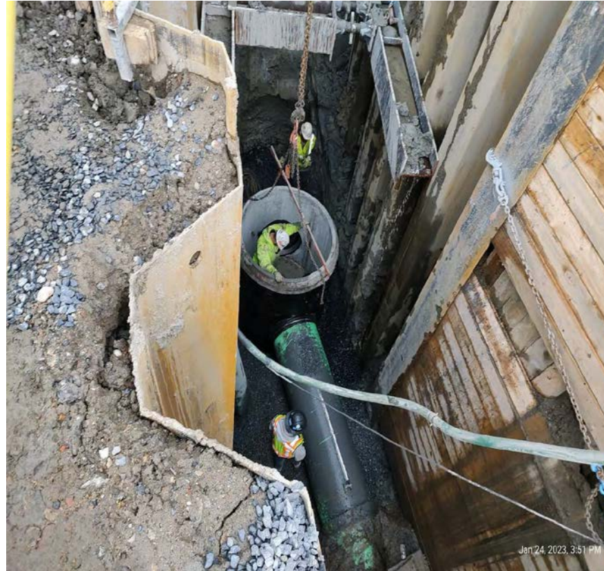
Manhole installation 1/24/23
