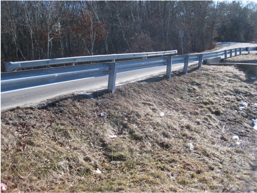
Figure 19. Unsupported Bridge Rail
