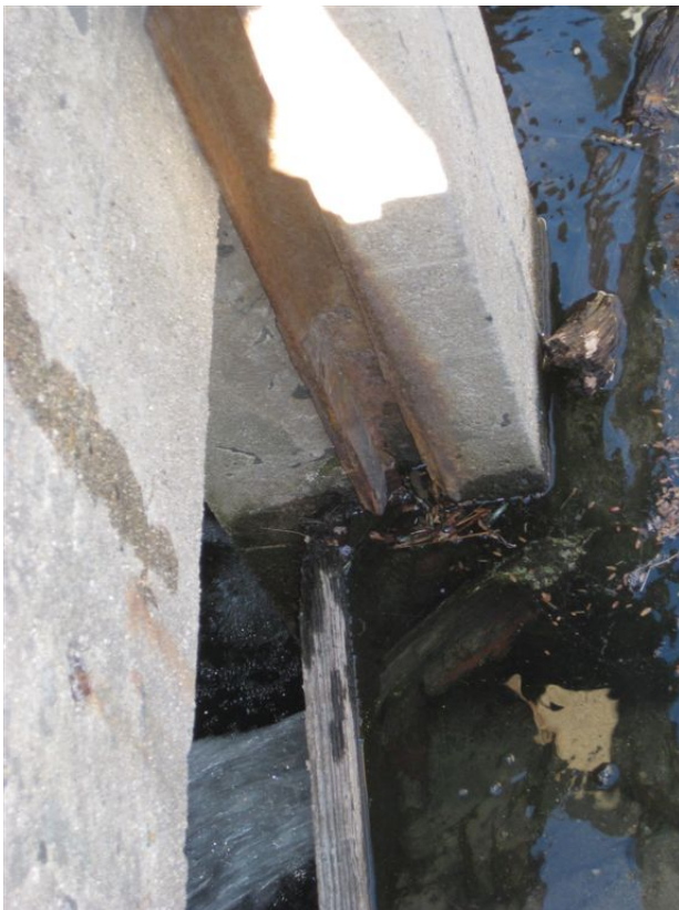
Figure 14. Misaligned Flash Boards
