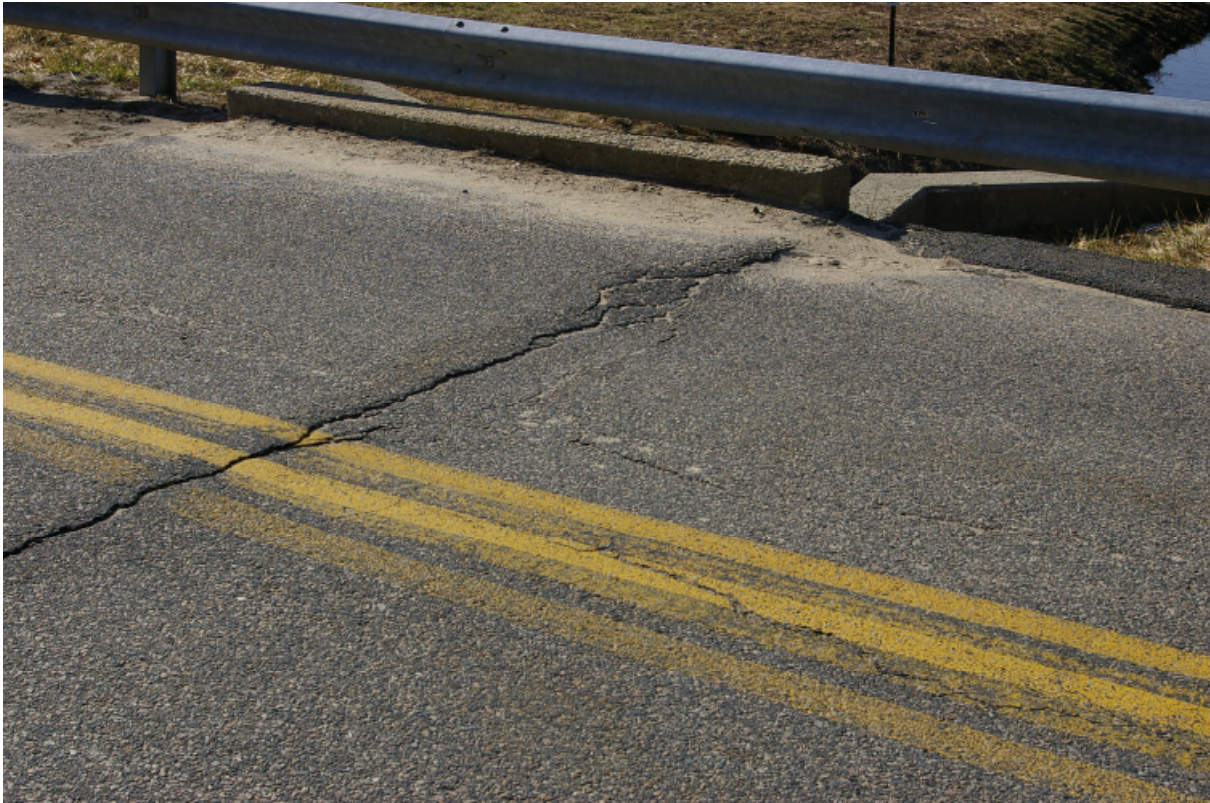
Figure 17. Settlement East Approach
