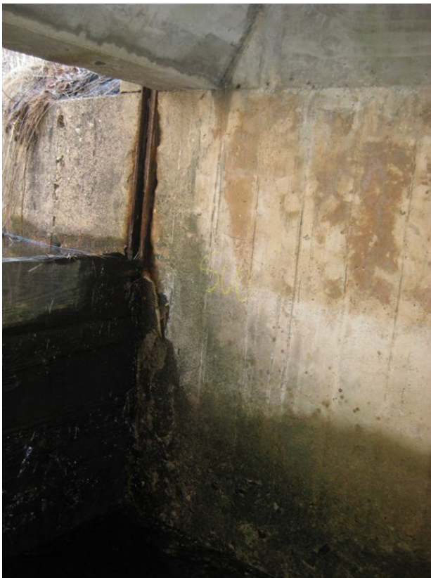
Figure 12. Scaling and Spalling West Breast Wall South End Bartlett Road over Beaver Dam Brook Plymouth, MA
