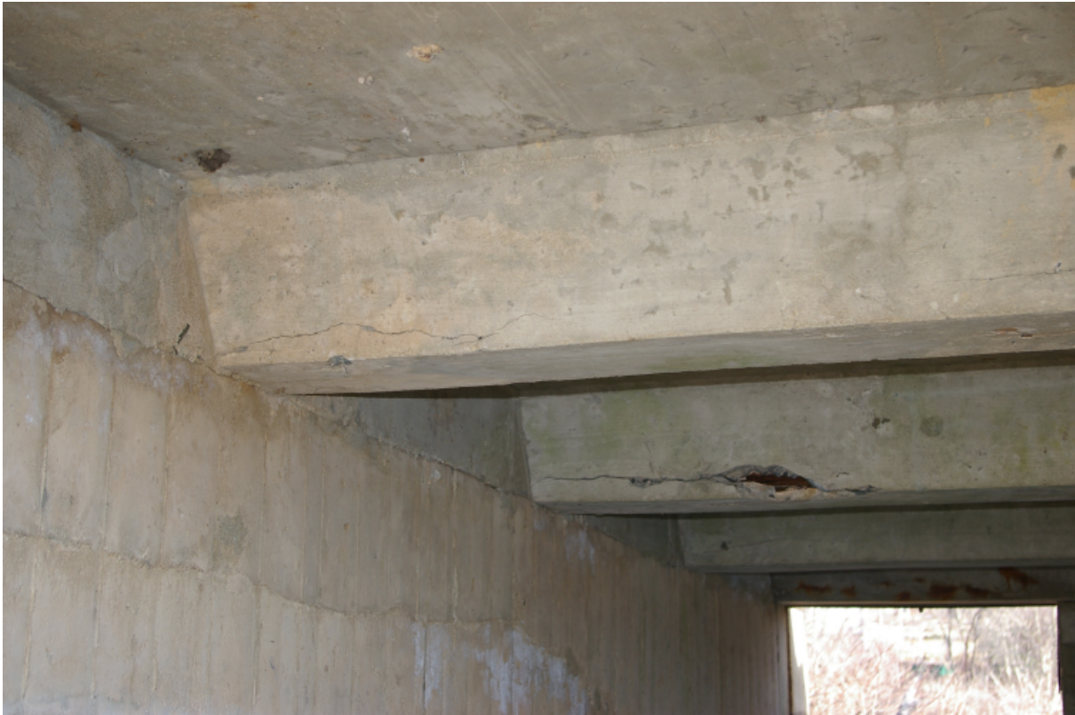
Figure 11. Delamination and Cracking Concrete Encasement
