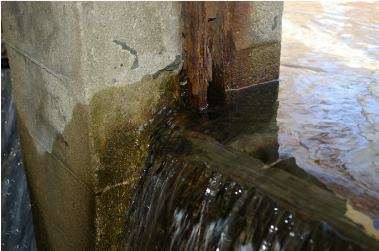
Figure 13. Misaligned Flash Boards
