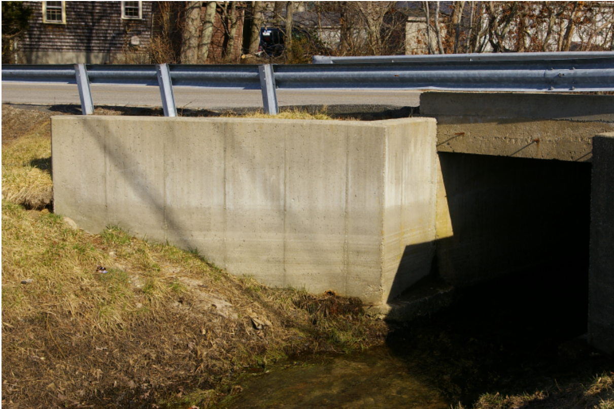
Figure 9. Northeast Wing Wall
