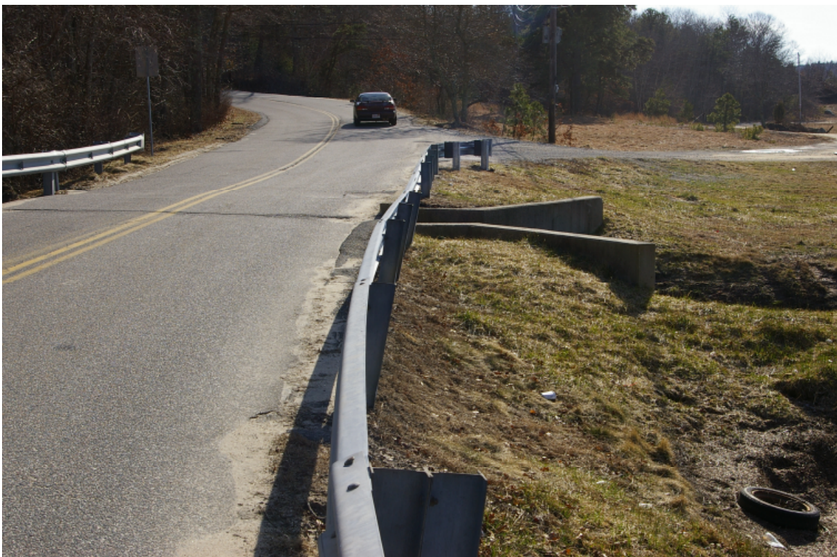
Figure 20. Misaligned Bridge Rail
