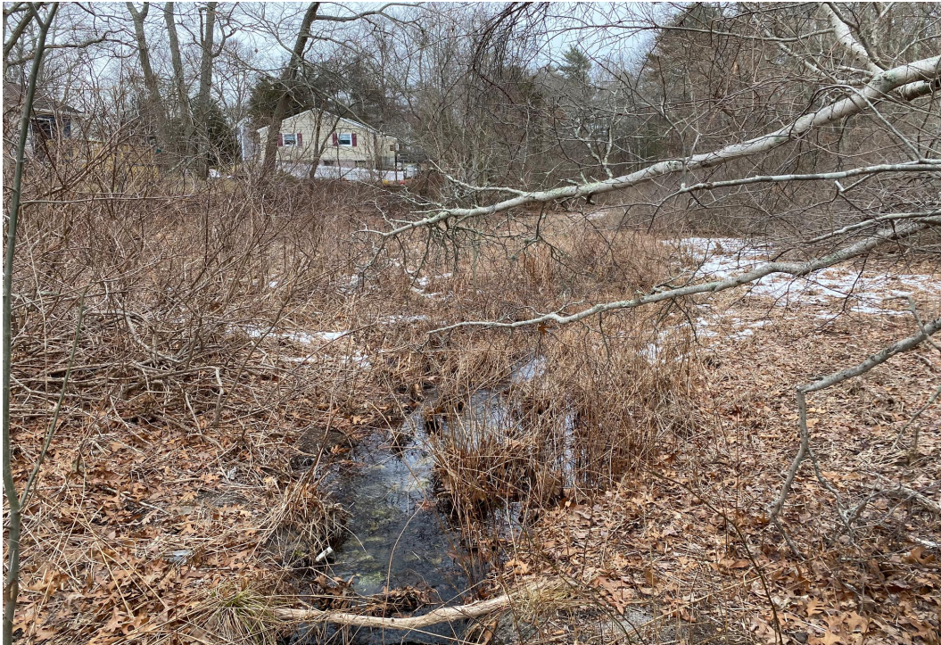
Upstream of Bridge/Culvert
