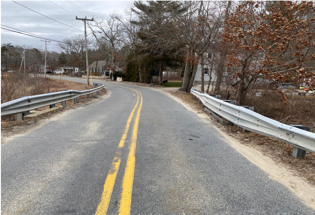
Bartlett Road over Beaver Dam Brook
