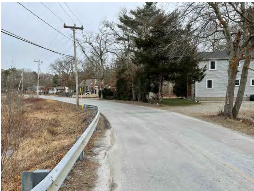
7 LOOKING NORTH @ BRIDGE
