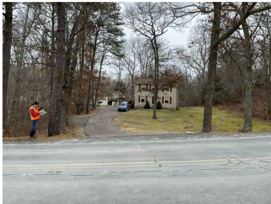
5 DRIVEWAY TO BE RECONSTRUCTED
