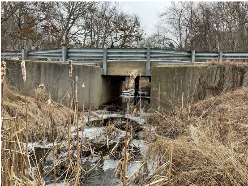
2 DOWNSTREAM ELEVATION (LOOKING UPSTREAM)
