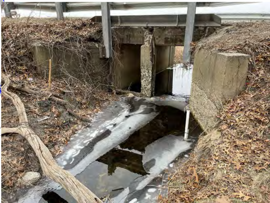
4 UPSTREAM ELEVATION (LOOKING DOWNSTREAM)
