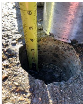
Photo 1. 4” Diameter Concrete Core, Above Beam 8, 12” From Face of West Abutment
