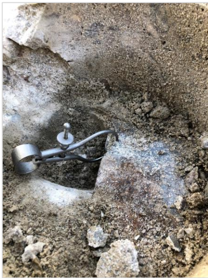
Photo 3. Flange Thickness Measurement
