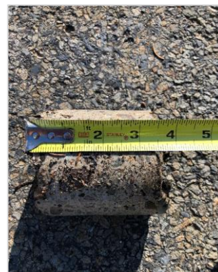
Photo 2. 4” Diameter Concrete Core, Above Beam 8, 12” From Face of West Abutment
