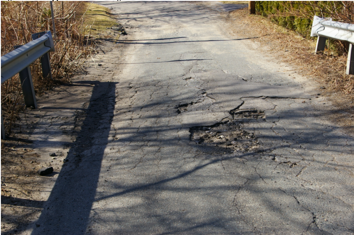
Figure 17 Pavement Failure West Approach
