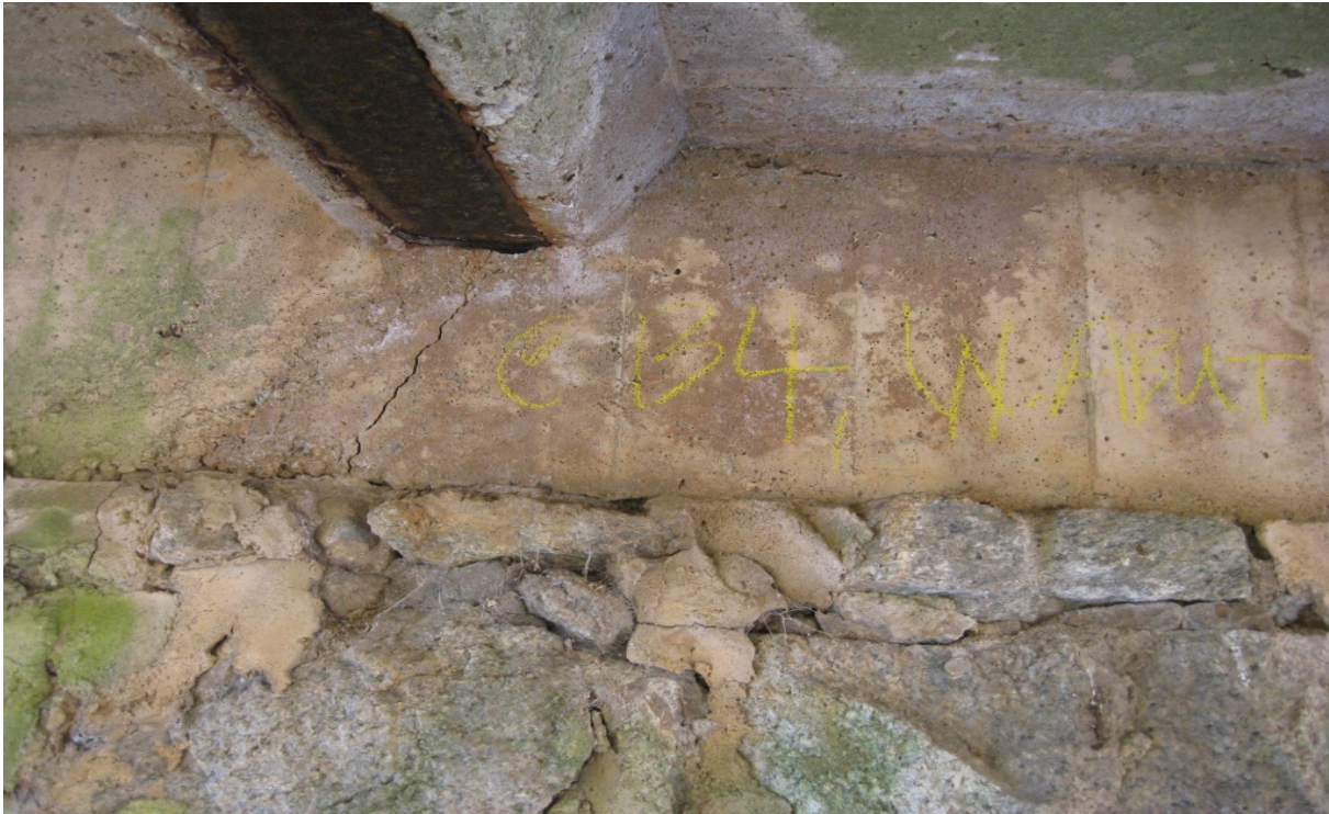
Figure 9 Crack in West Abutment Bridge Seat (below girder 4)
