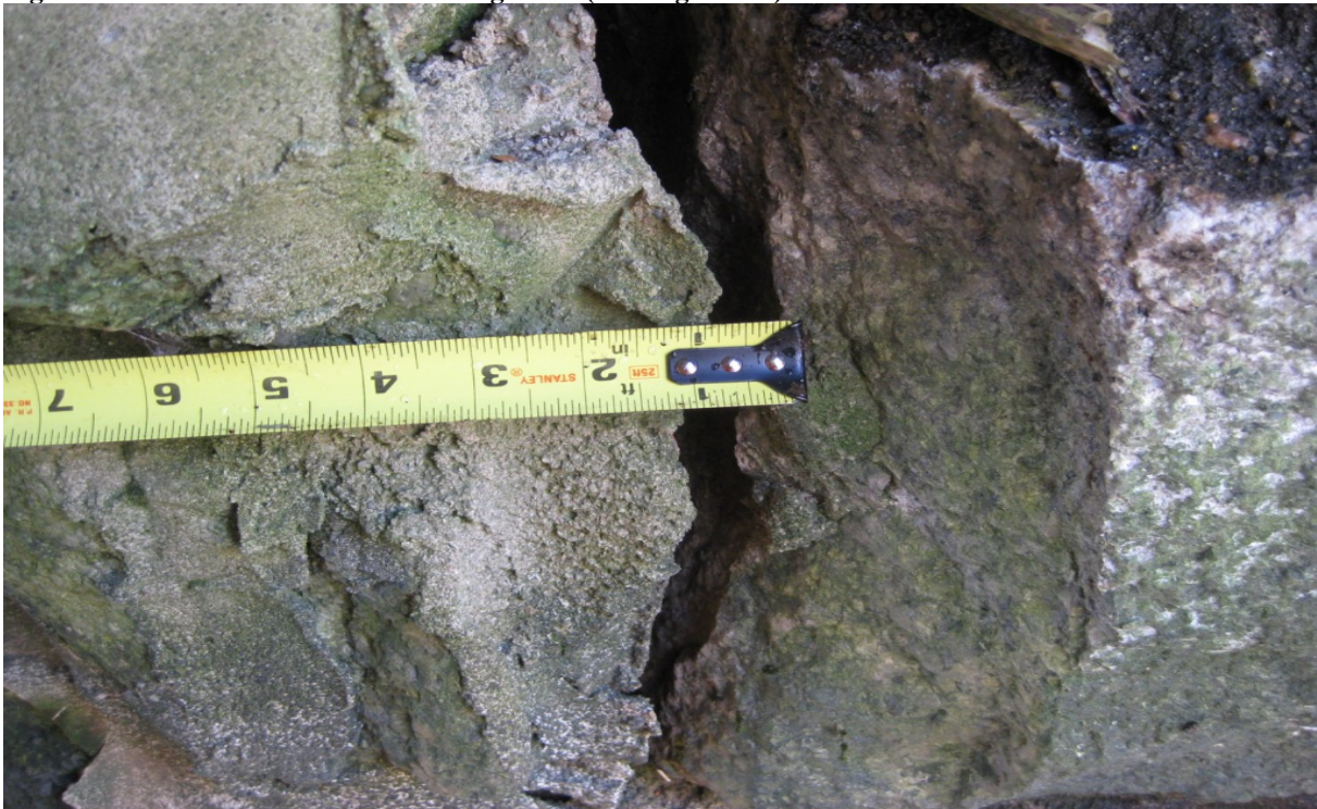
Figure 10 Lateral Displacement North End West Breast Wall
