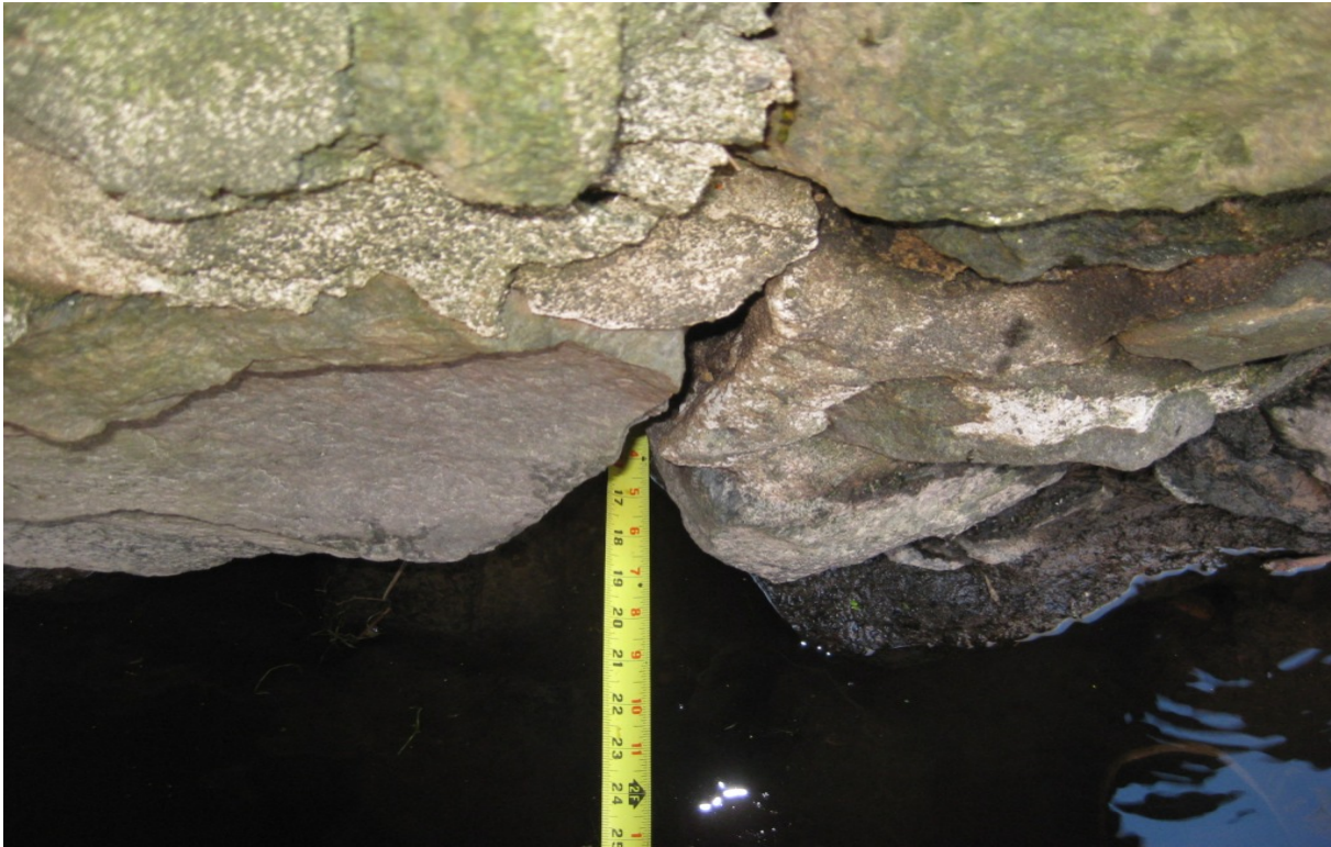
Figure 12 Void West Breast Wall
