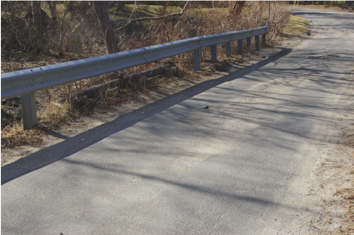
Figure 16 Unsupported South Bridge Rail
