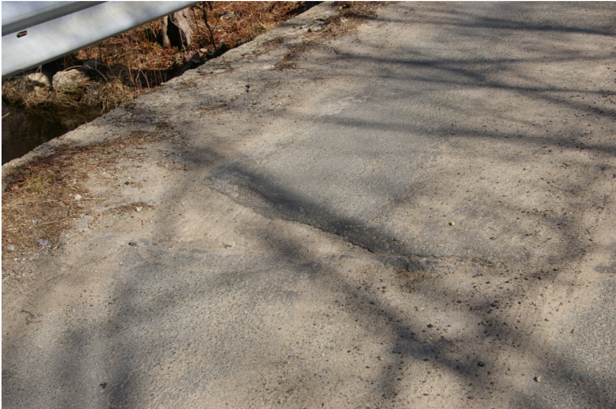
Figure 18 Settlement North Side West Approach
