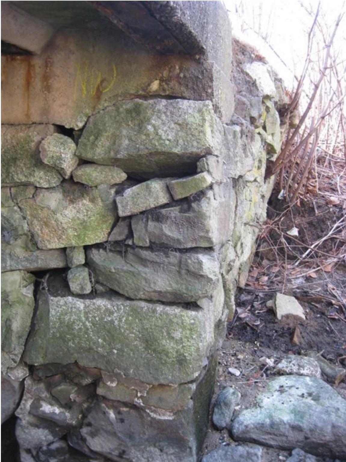
Figure 11 Settlement and Lateral Movement North West Wing Wall
