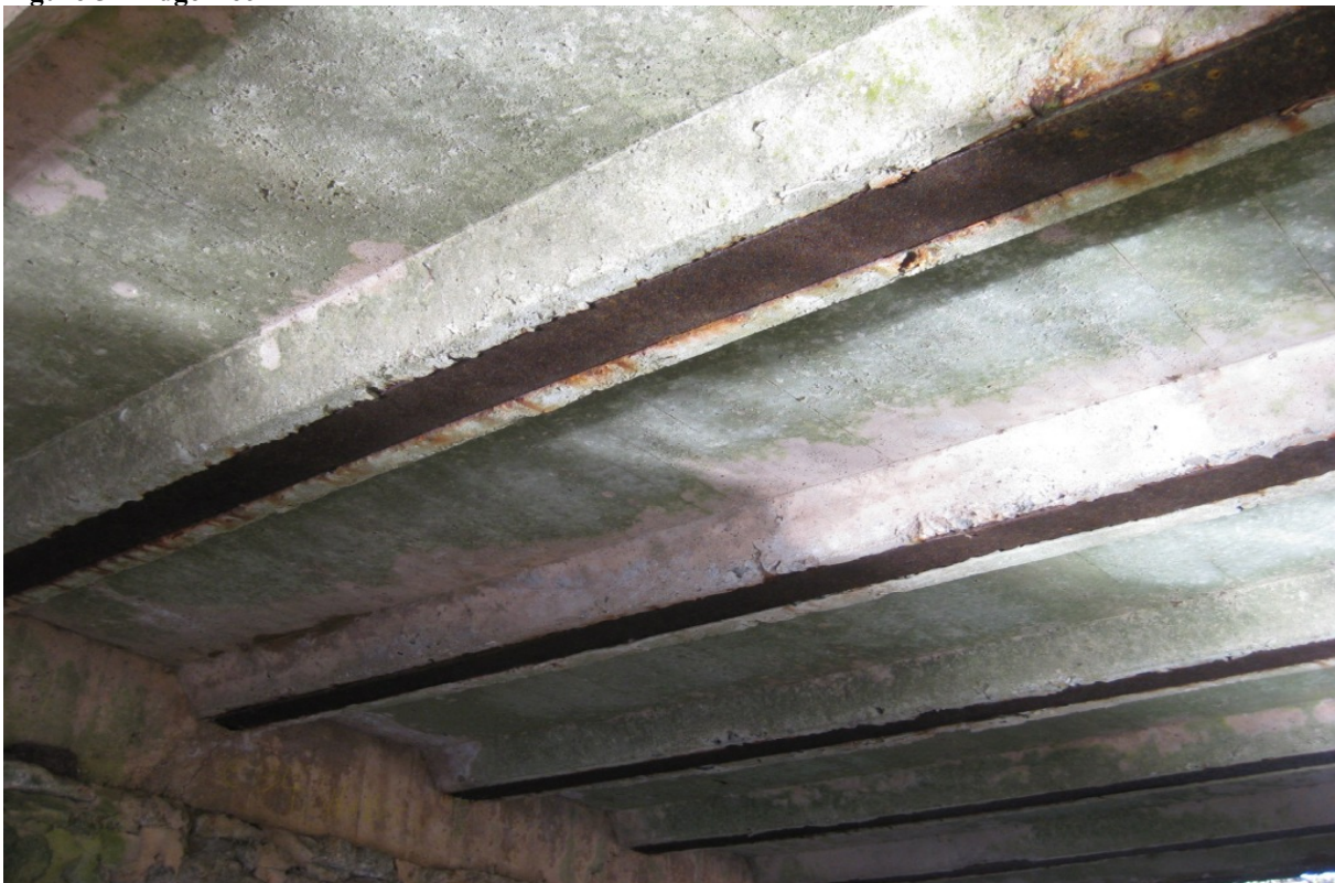
Figure 6 Girders (viewed from underside of bridge deck)
