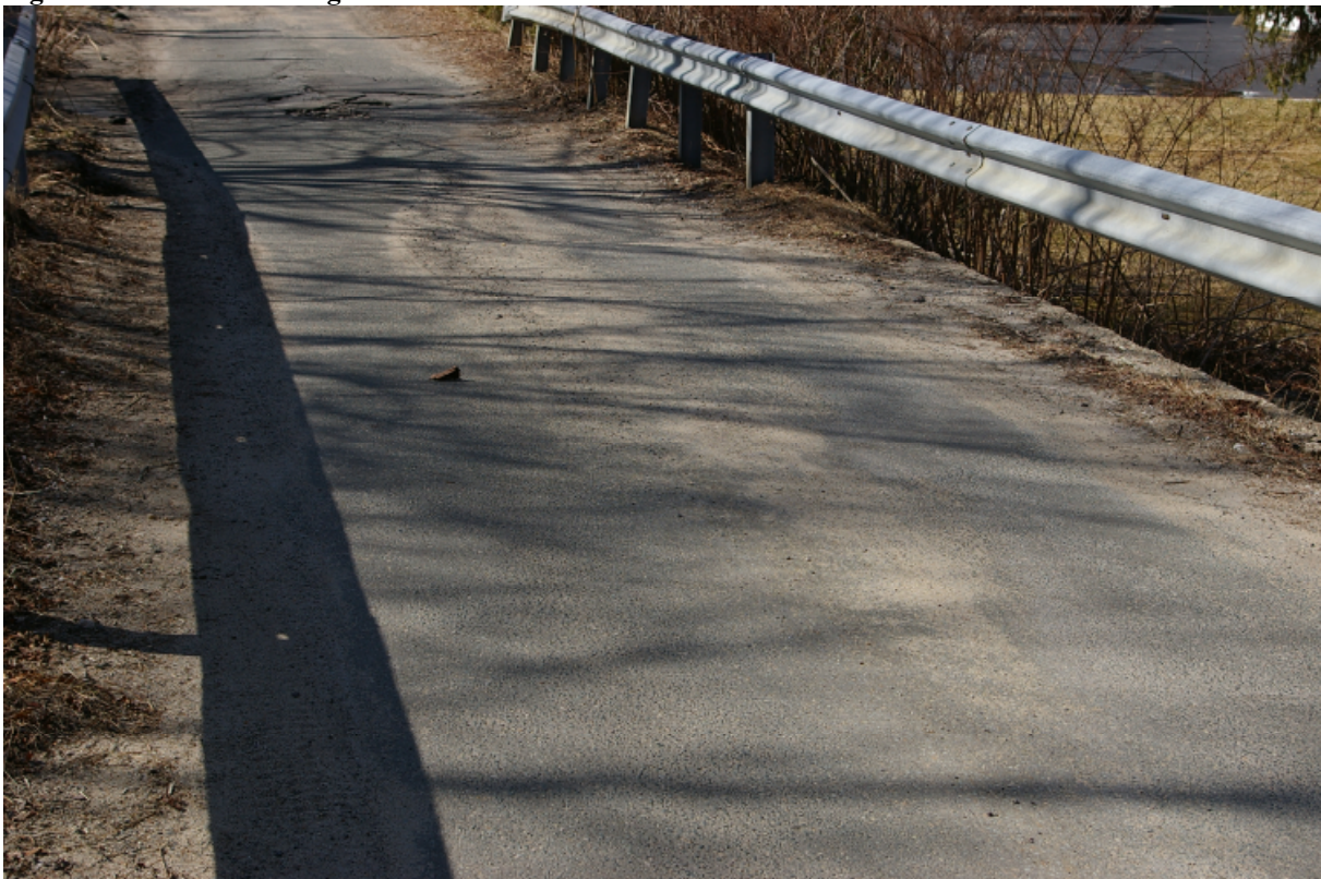
Figure 15 Unsupported North Bridge Rail
