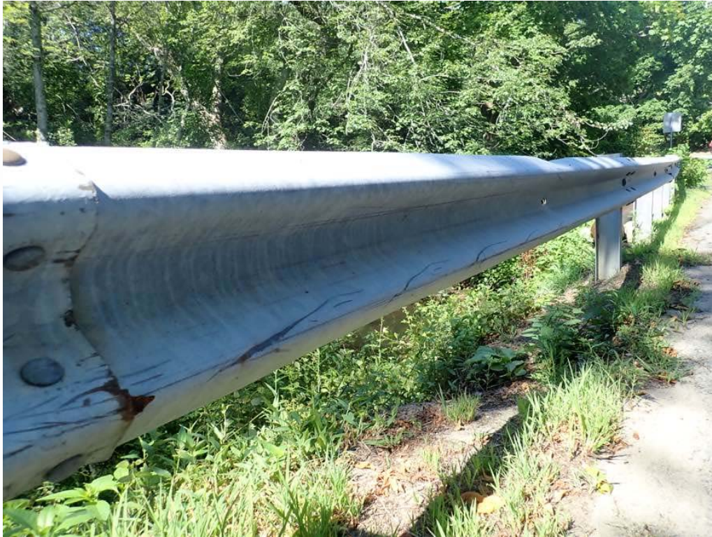
Photo 7: South rail minor collision damage scrapes.
