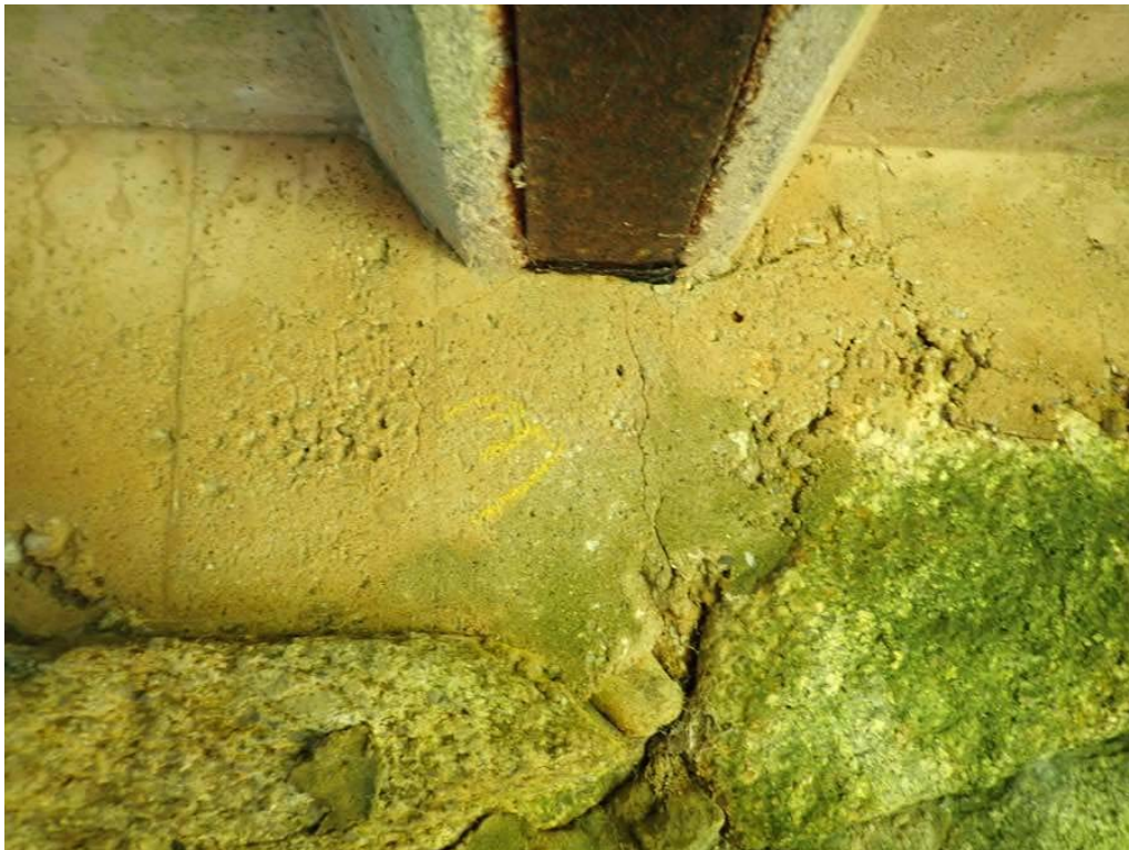
Photo 16: East abutment below beam 3 hairline vertical crack.
