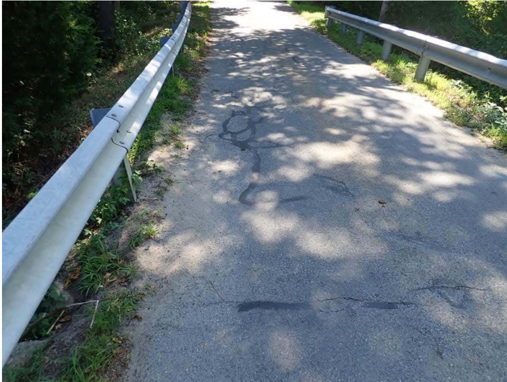
Photo 11: East approach looking east sealed and unsealed longitudinal cracking.
