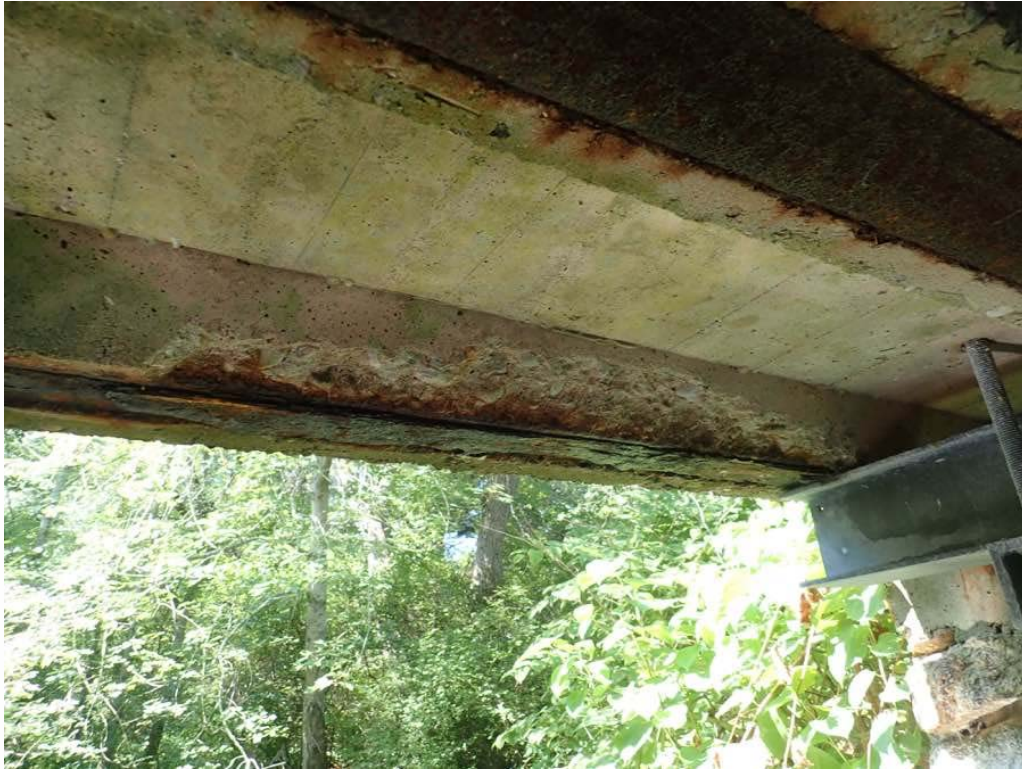
Photo 3: Beam 1 south elevation spall.
