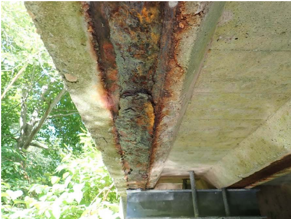
Photo 12: Beam 1 looking west from midspan, section loss.
