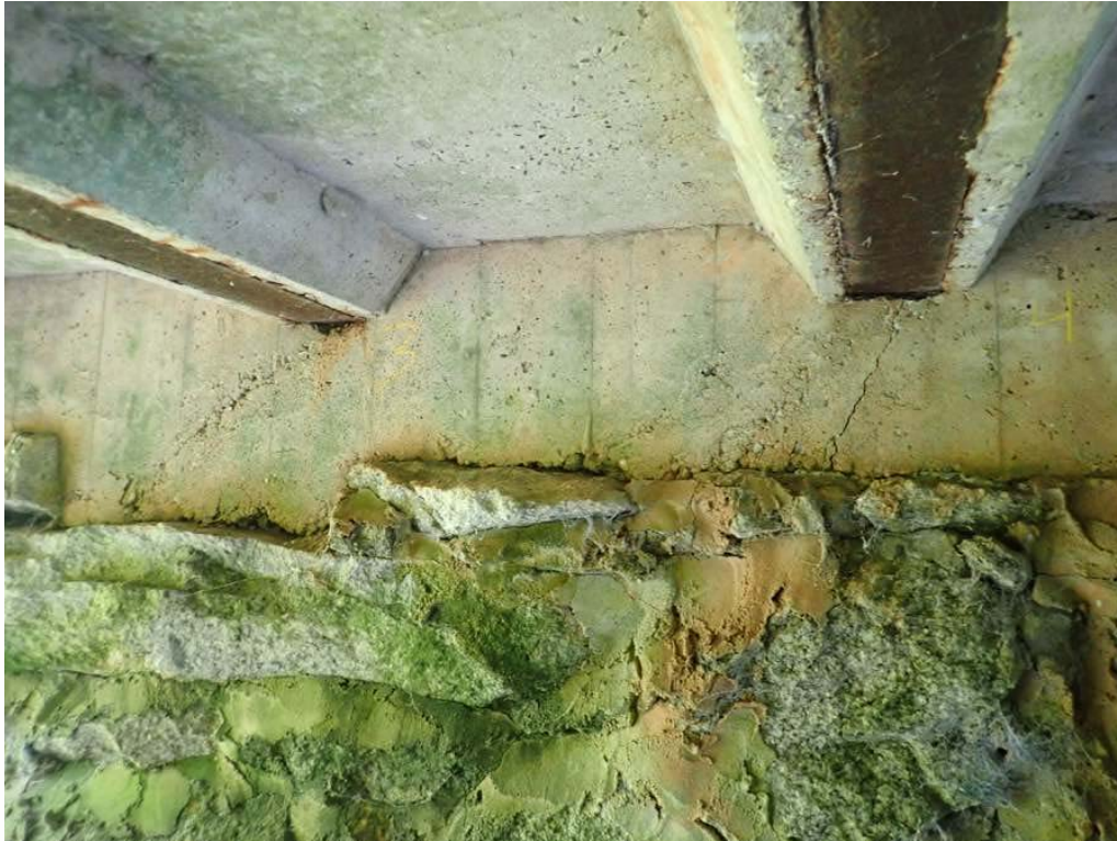
Photo 15: West abutment below beam 3 & 4, honeycombing and cracking.
