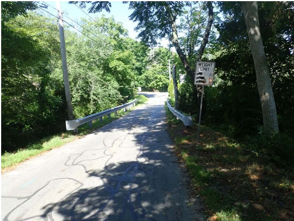
Photo 10: East approach sealed and unsealed cracking.
