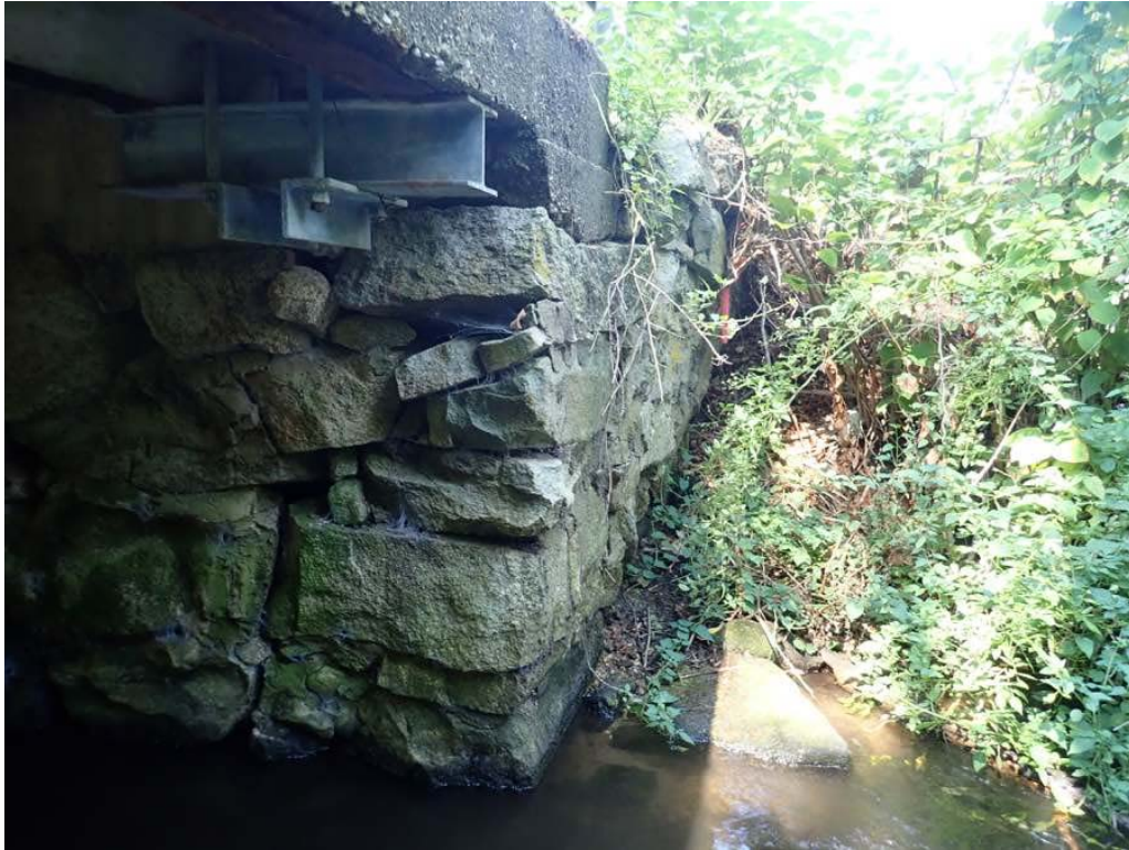
Photo 19: Northwest wingwall leaning and voids in breastwall.
