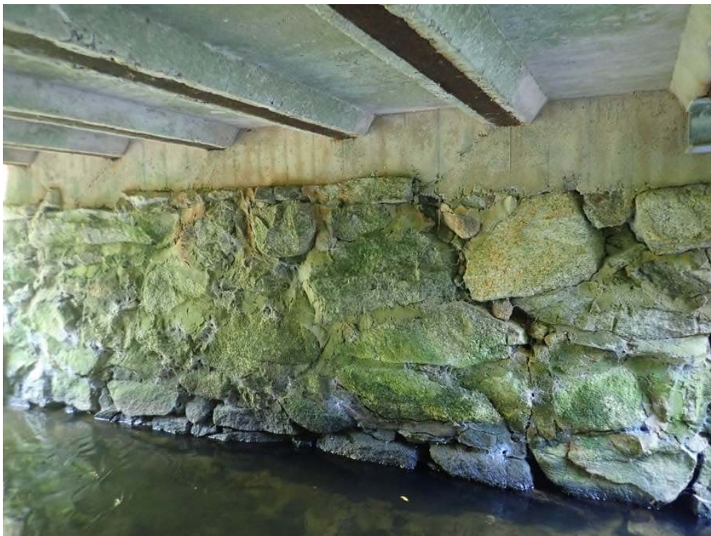
Photo 18: West breastwall overview voids.
