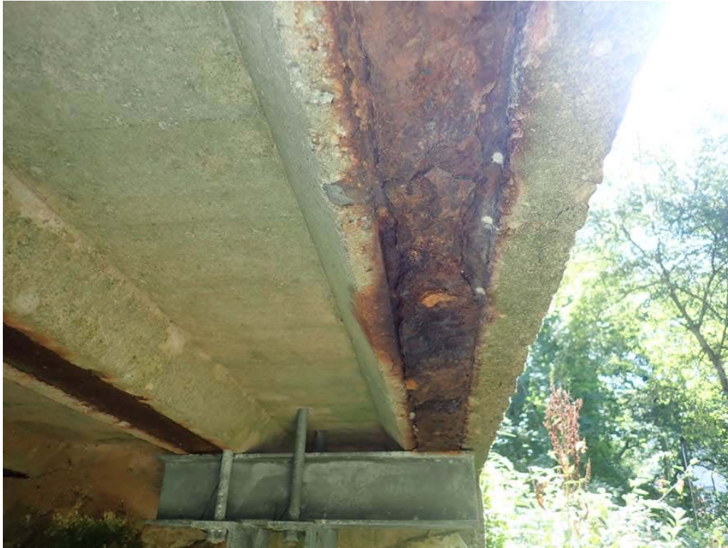
Photo 13: Beam 1 looking east from midspan, section loss.
