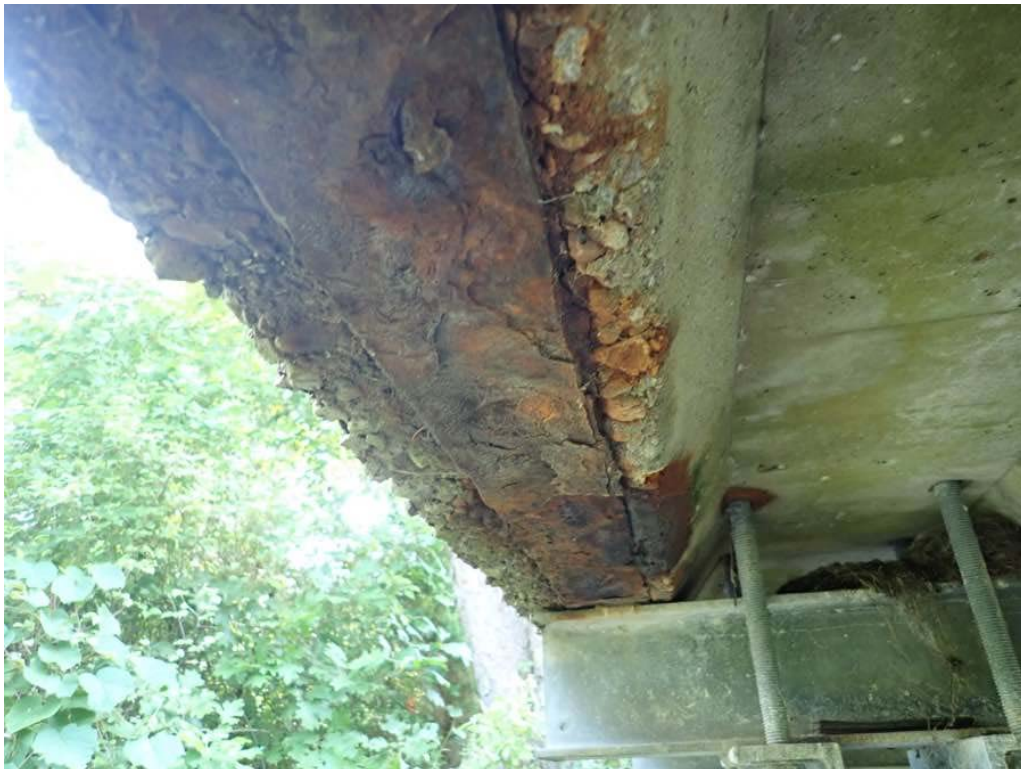
Photo 14: Beam 8 looking east pitting.
