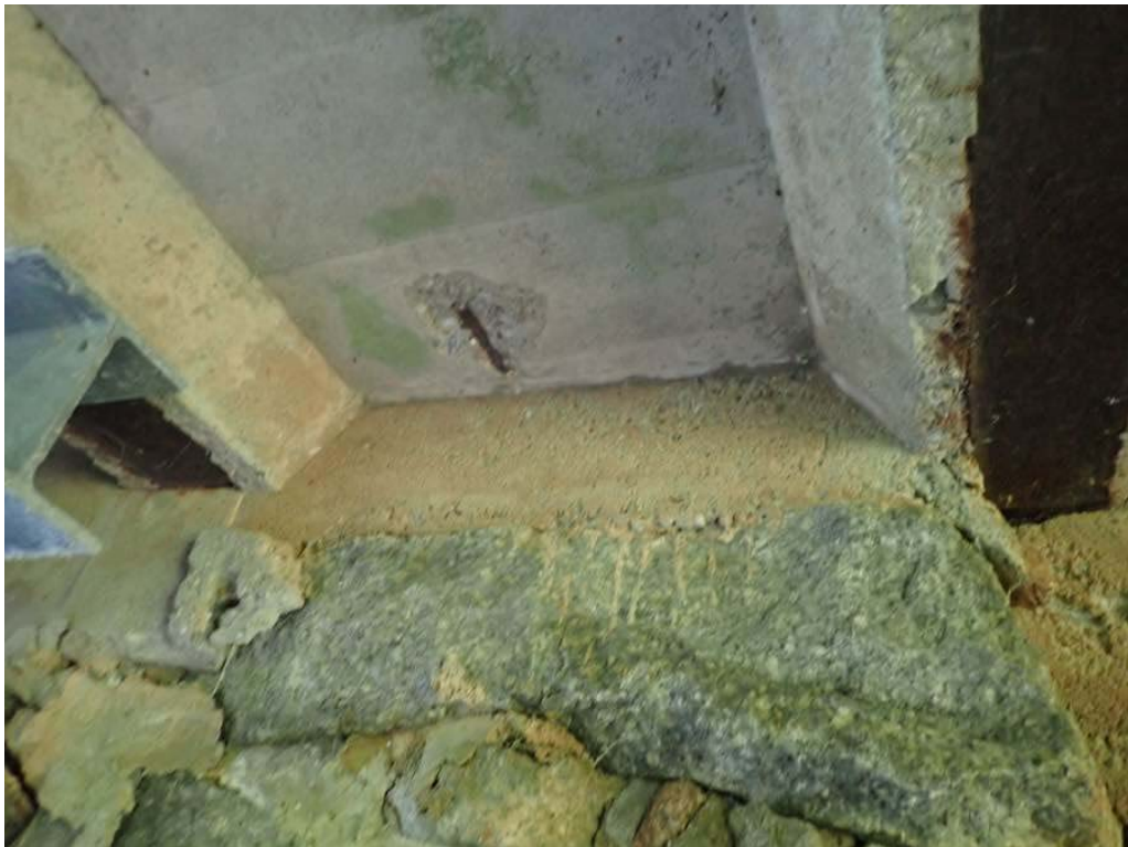
Photo 6: Bay 6 at east abutment minor spall.
