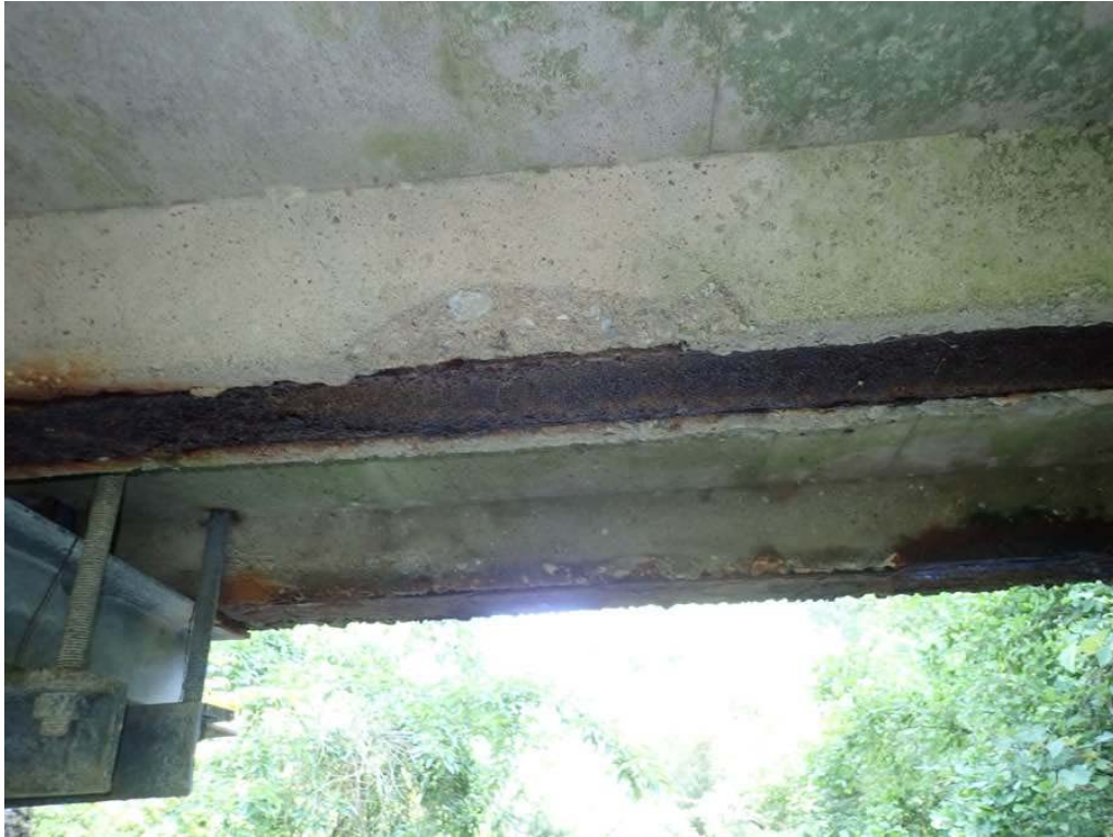
Photo 5: Beam 7 near west abutment spall.
