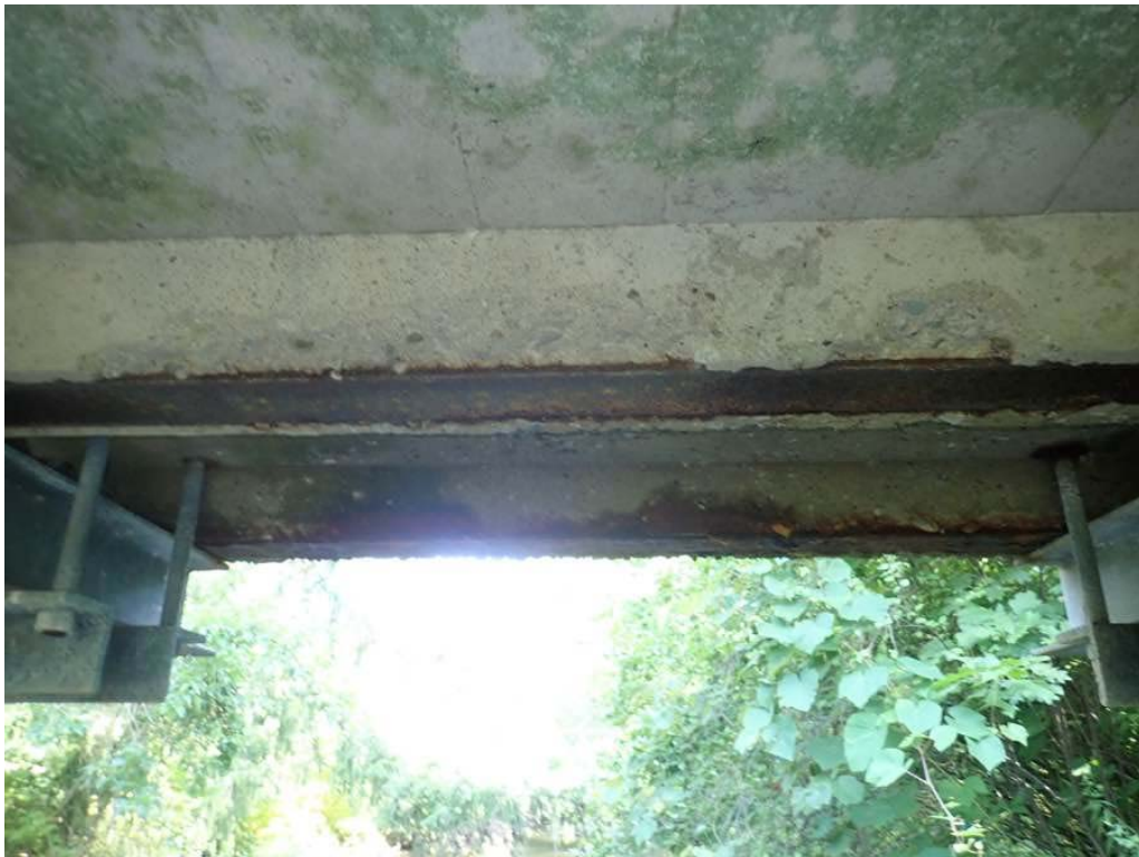
Photo 4: Beam 7 south elevation near east abutment spall.
