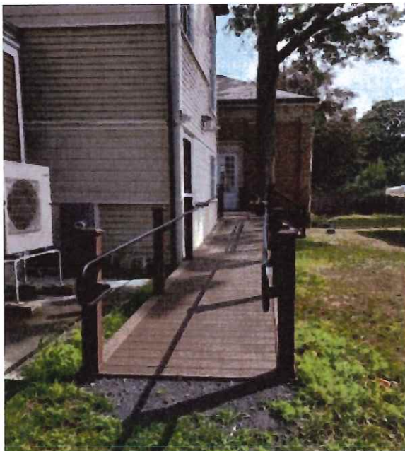
Rear Accessibility Ramp – Needs Cement Pad Landing
