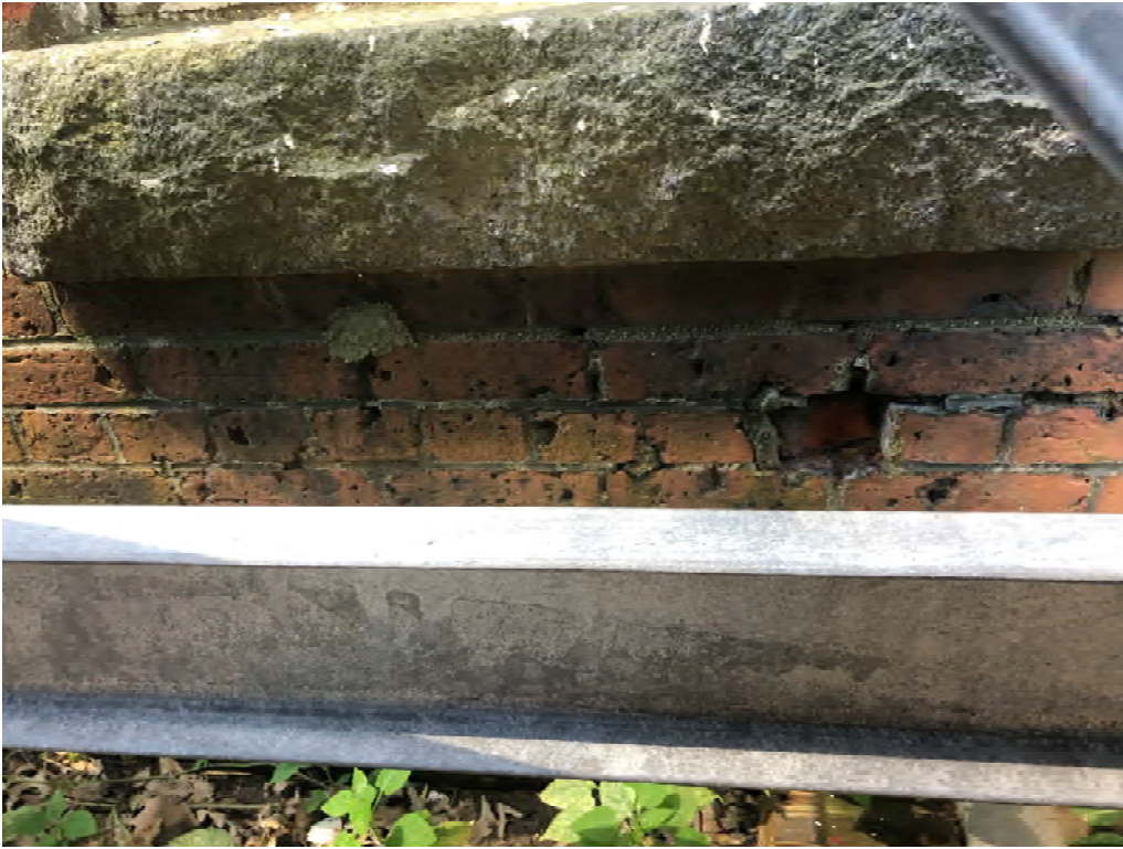
Figure 2: North elevation, damaged/missing brick.
