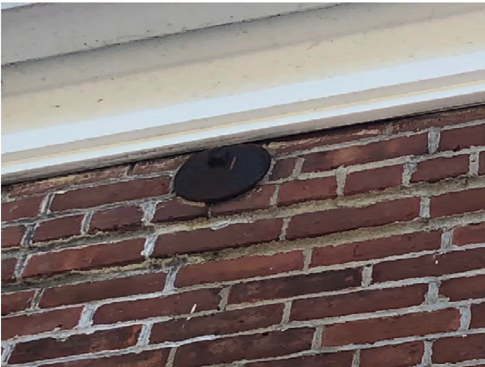
Figure 5: Tie rod at west elevation.
