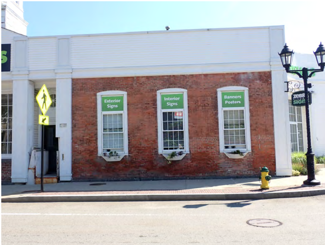
Figure 14: West elevation, south end; replacement windows set in masonry openings.
