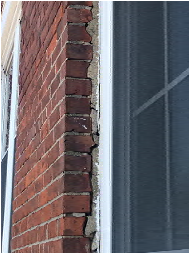
Figure 4: West elevation (front); slight movement of wall at jamb, allowing for water to enter into the wall.
