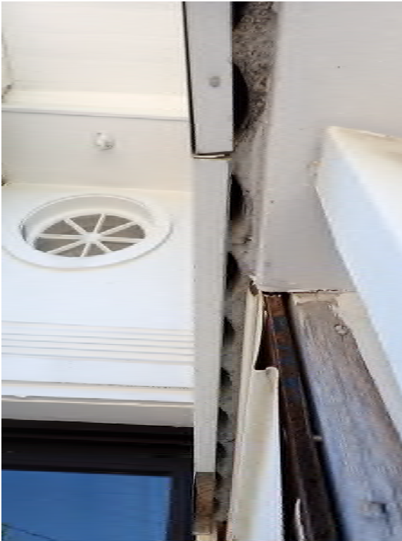
Figure 19: West elevation, evidence of original wood fluted pilaster beneath aluminum siding.
