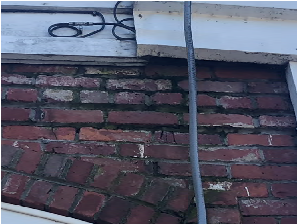
Figure 10: North elevation, heavy biological growth, particularly at mortar joints.
