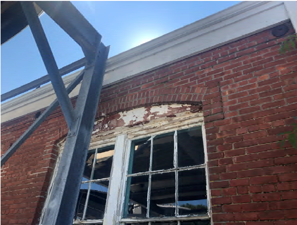
Figure 17: 2 nd window bay of north elevation, original wood window that may predate 1940's work.
