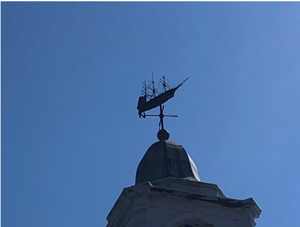
Figure 23: Original weathervane, missing directionals "S" and "W".
