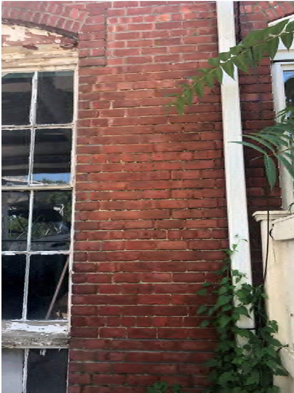
Figure 7: North elevation, typical deteriorated mortar joints.
