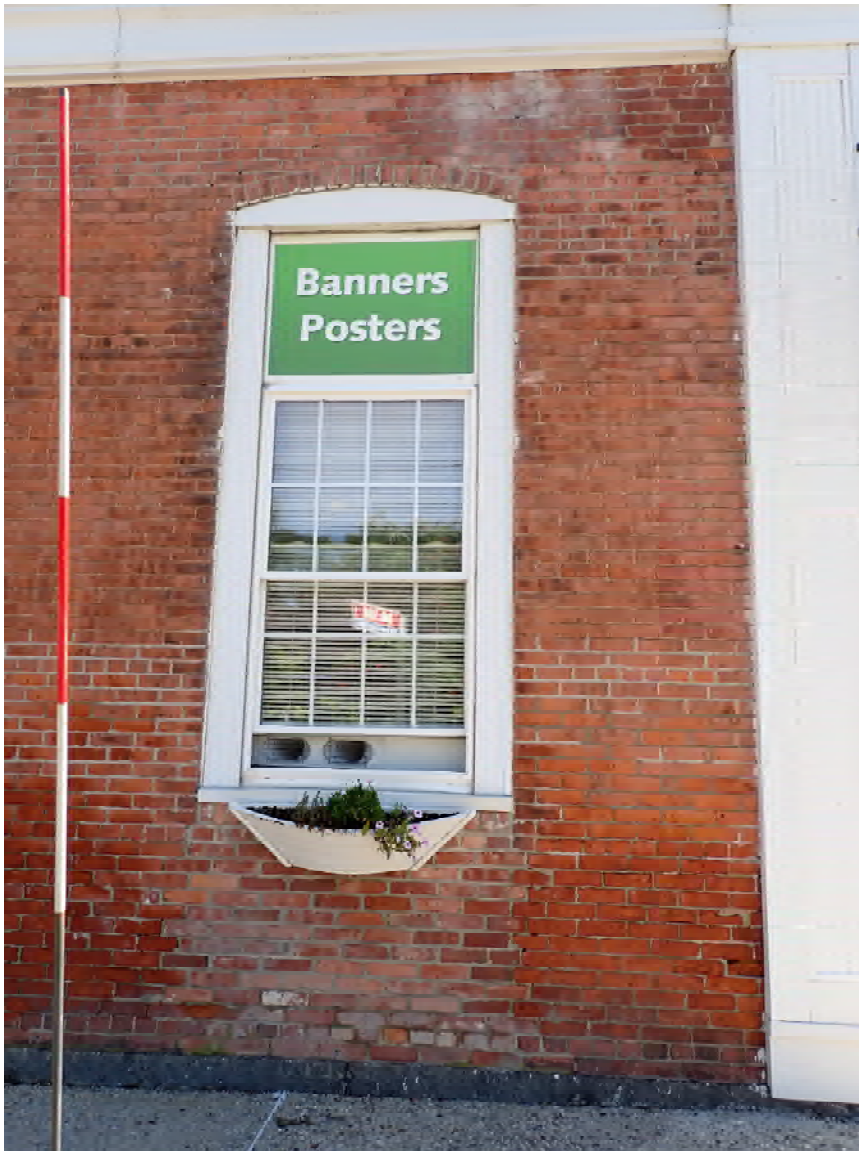
Figure 12: West elevation, paint haze and efflorescence on brick.
