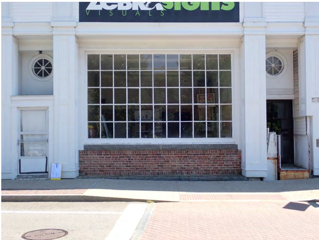
Figure 15: Wood windows dating to 1940's, including central bay window and side circular windows.
