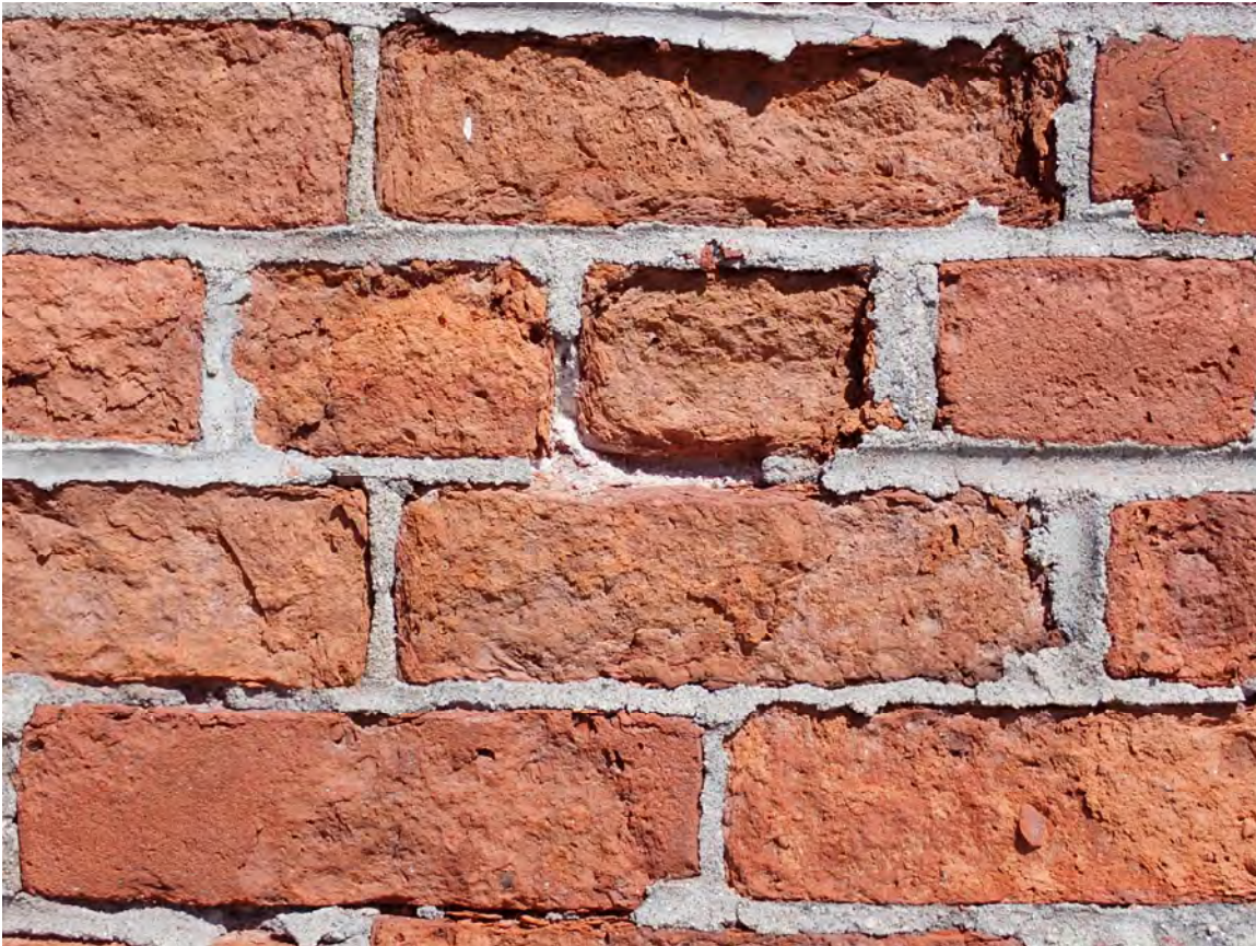
Figure 1: South elevation, west end. Brick laid in English bond with red brick. Spalled brick caused by repointing mortar that is too hard and not compatible with the soft brick.
