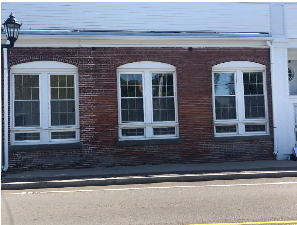
Figure 8. West elevation; poorly color matched and installed repointing mortar.
