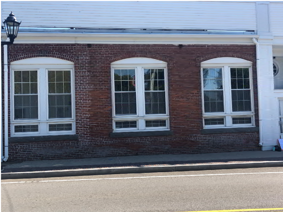
Figure 13: West elevation, north end; replacement windows set in masonry openings.
