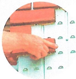
Mounting Glen-Gery thin brick to Thin Tech panel (Elite).
