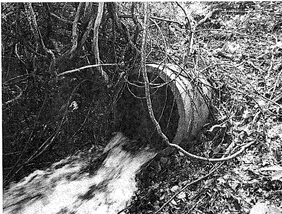
Photo 18: View of 30" RCP outlet into Hedges Pond, facing west.
