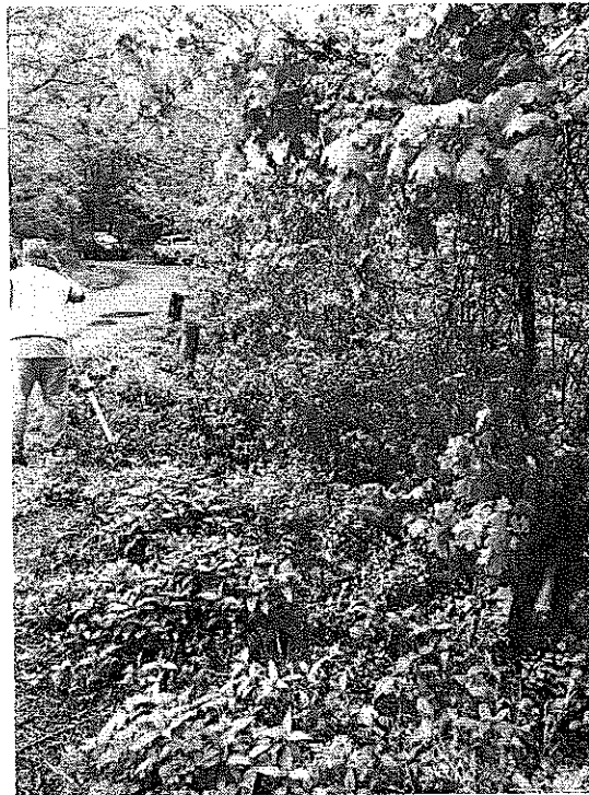
Photo 14: View of downstream slope taken from the right embankment, facing northwest; note overgrown vegetation.
