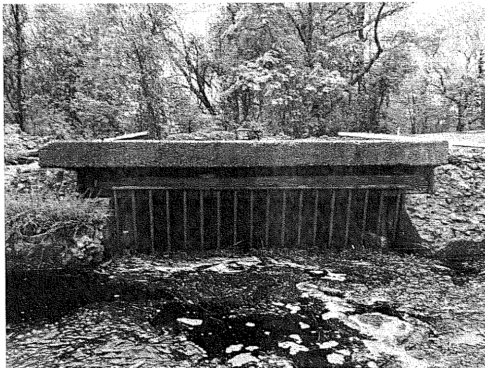
Photo 8: View of drop inlet spillway with trash rack, facing northeast; note concrete spalling and debris buildup in front of the trash rack.
