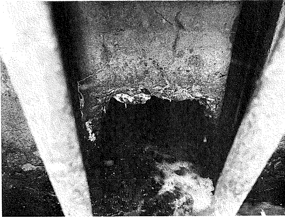
Photo 11: View of 30" diameter steel outlet pipe from the drop inlet.
