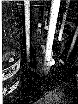
Heating Plant Chemical Shot Feeder
