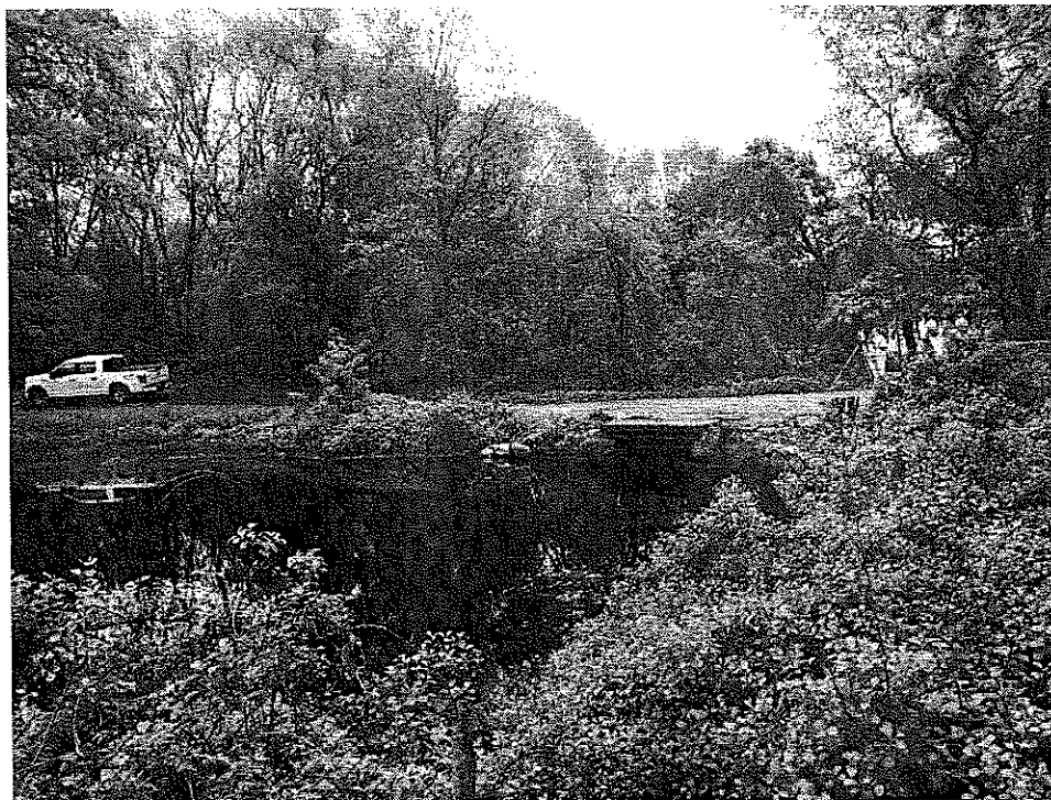
Photo 6: Overview of the upstream slope taken from the right shoreline, facing north; note overgrown vegetation on the slope and right abutment.
