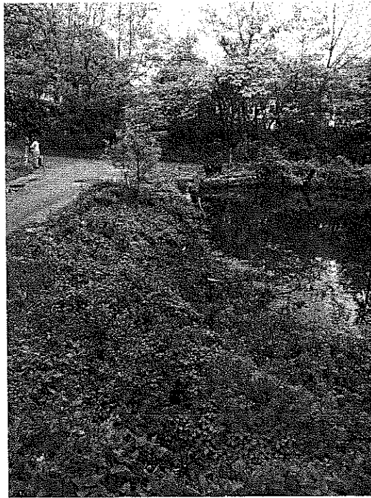
Photo 7: View of upstream slope taken from the left abutment, facing southeast; note overgrown vegetation.
