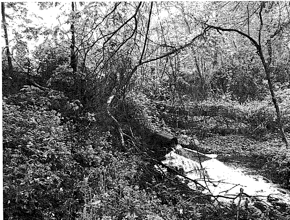
Photo 16: View of embankment downstream slope and discharge area, facing west; note large downed tree at mid-slope and 12" steel outlet pipe.
