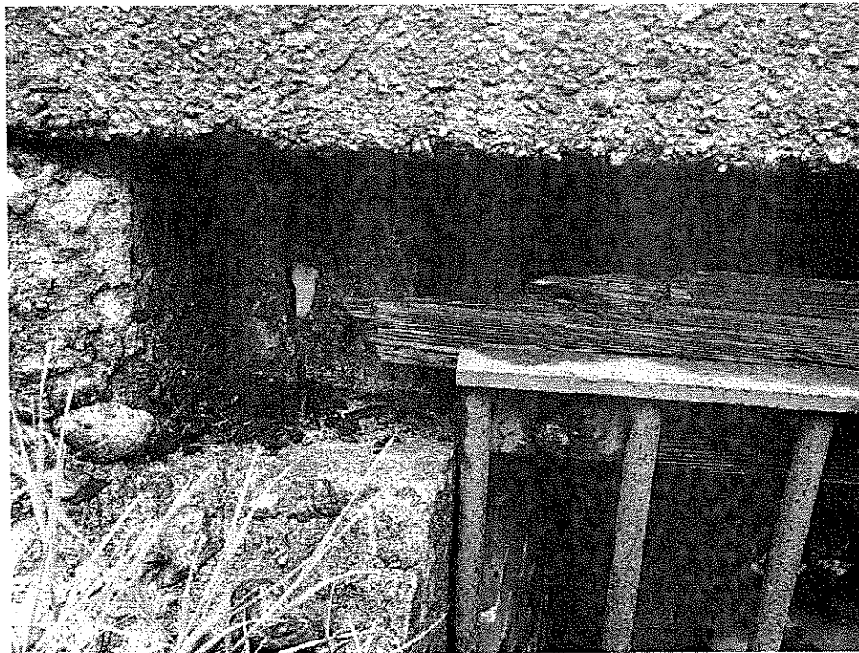
Photo 10: View of deteriorated trash rack and timber support beam at left side of spillway.
